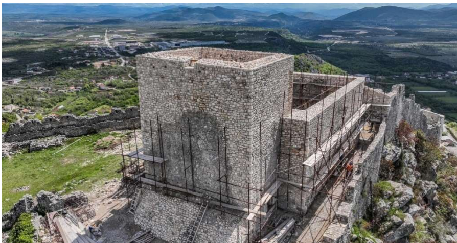
Figure 3. works on site
